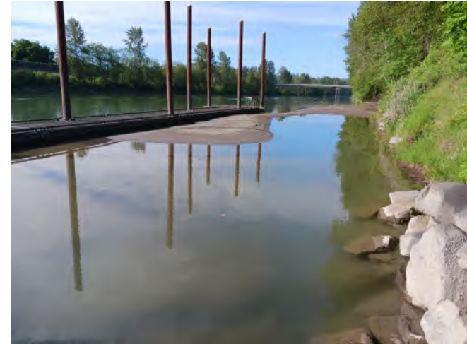
Photo 2. Taken June 2025. Looking downstream at dock shown in Photo 1. Both photos were taken at similar river levels. Photo 2 shows significant sediment accumulation.
